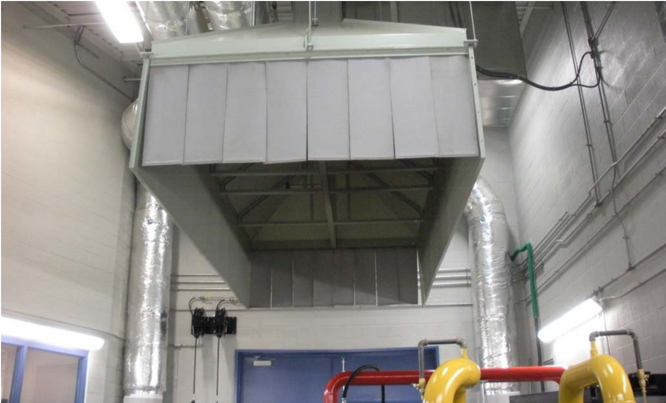
Illustration 58 – Exhaust Hood above Engine
